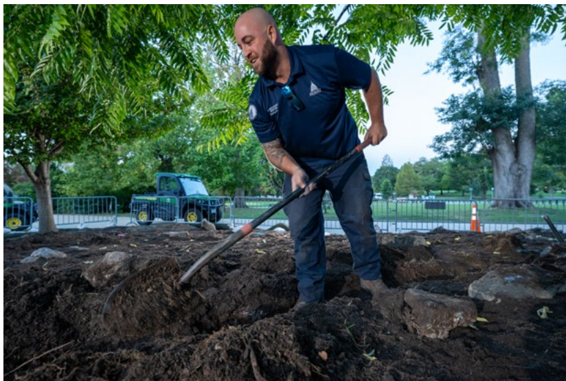
Pipefitter Adam McClanahan installs new irrigation for the planting beds.
