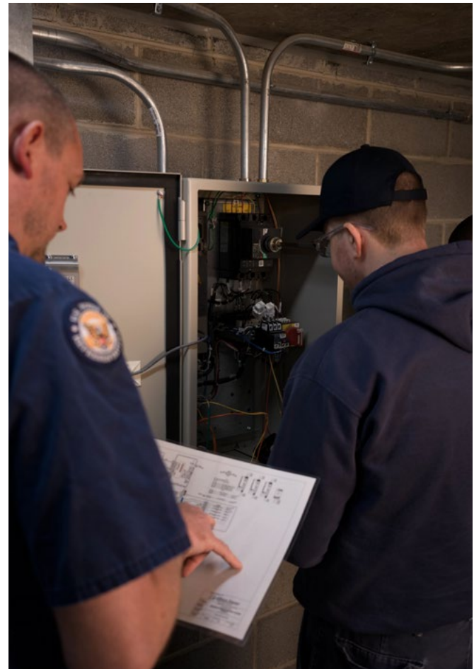
Day oversees Mullins' work on an HVAC control panel.
