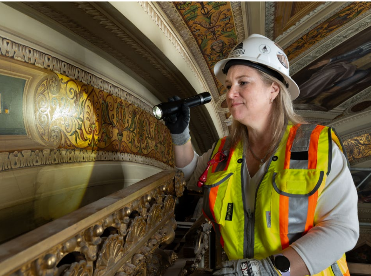
▼ Klee examines the recently surveyed Constantino Brumidi fresco in the President's Room in the U.S. Capitol dating from 1860. Recent surveys are assessing the condition of numerous painting media including fresco, tempera, oil on plaster and gilding.
