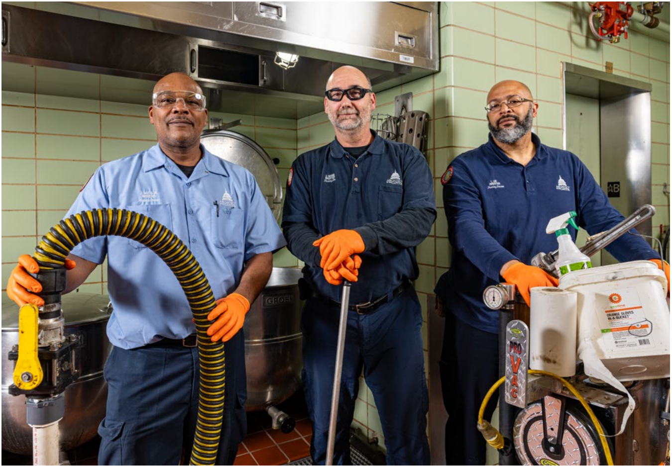
Capitol evening shift pipefitters, from left to right, John Watts, Dale Mathis and Lloyd Lee prepare to clean and maintain a kitchen drain interceptor system.
