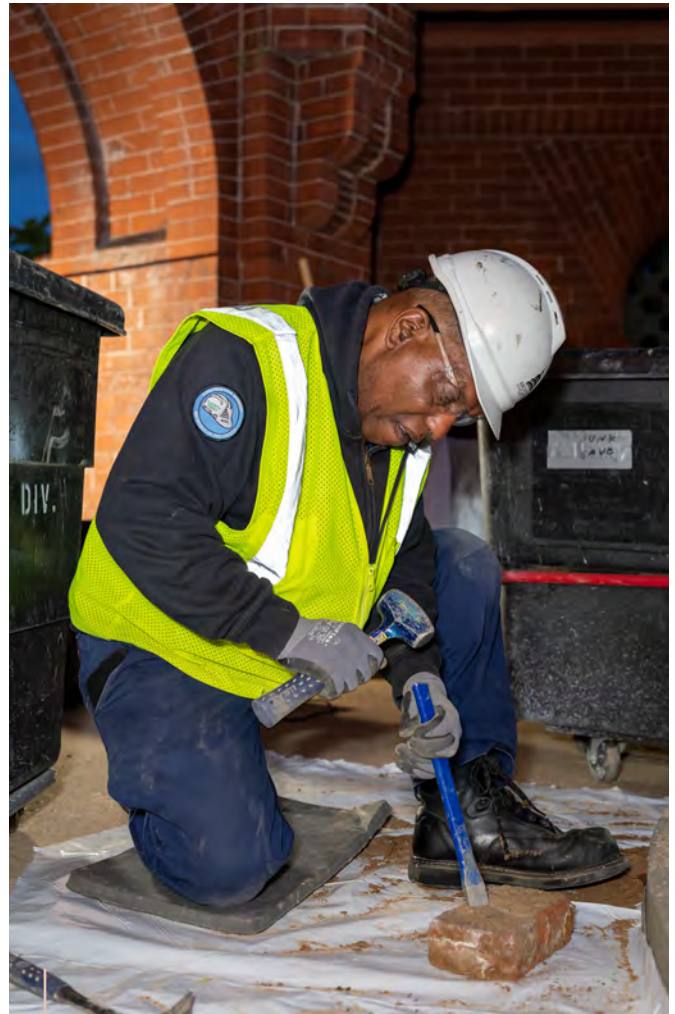
An AOC employee works on the repairs at the Summerhouse Fountain.
