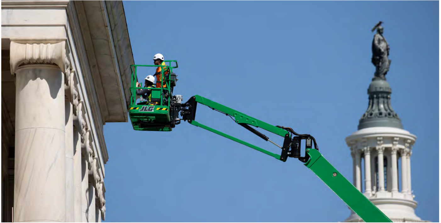
Stonework conditions surveys help the AOC assess future stonework preservation needs.
