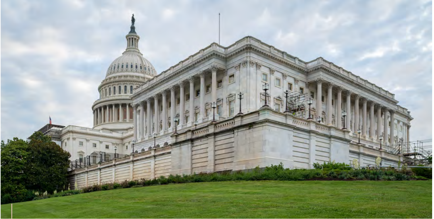
The south Olmsted Terrace wall encircles the U.S. Capitol where stonework projects continued in FY 2023.
