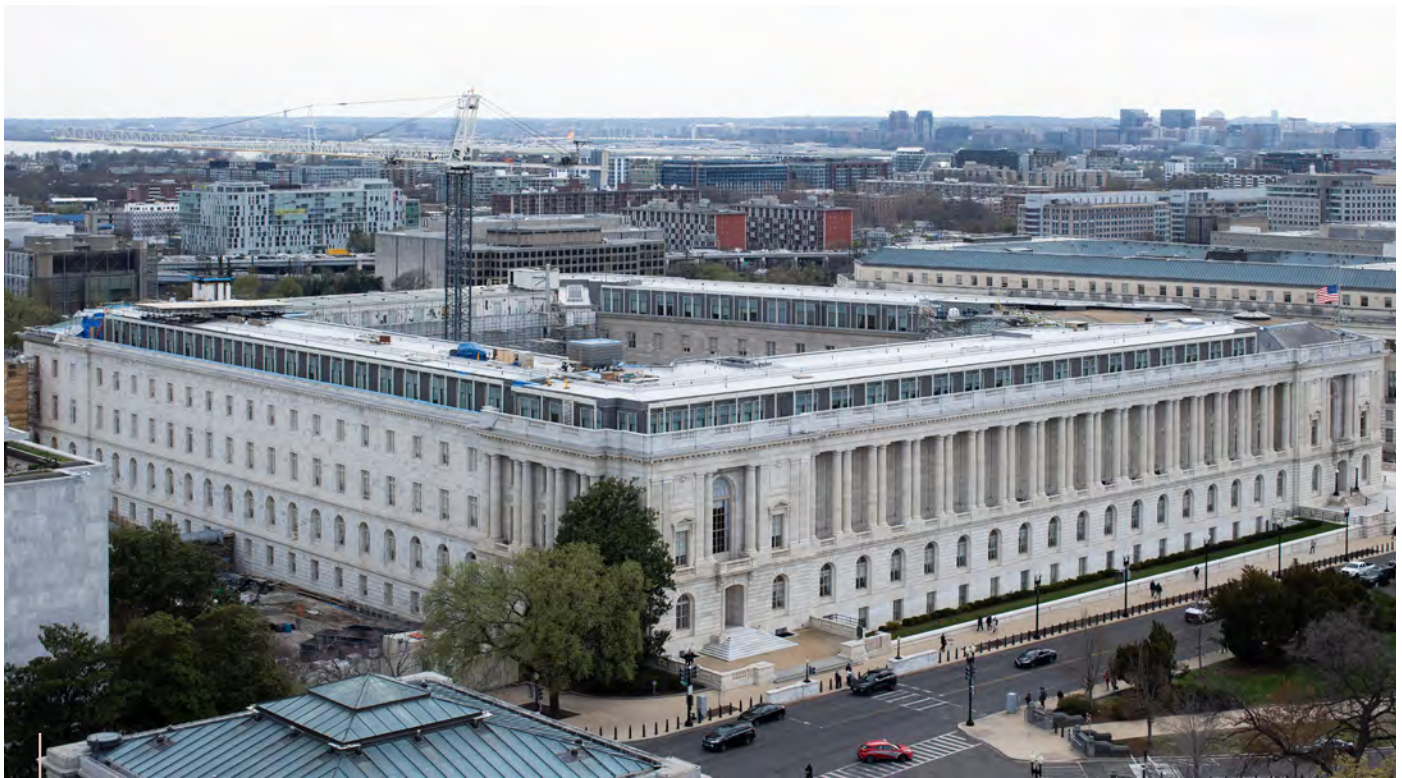
Phase 3 of the Cannon Renewal Project was completed in FY 2023.
