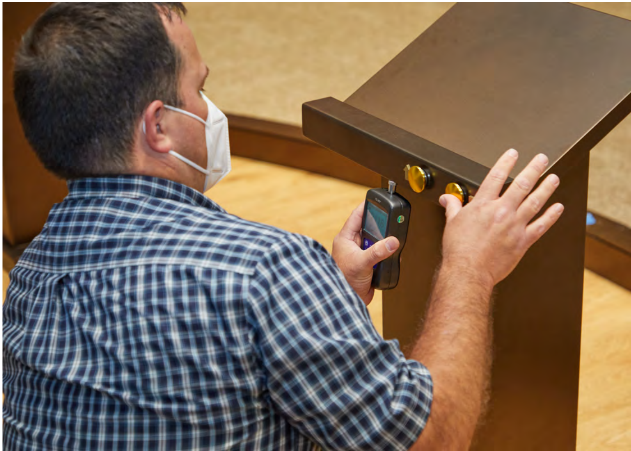
▼ AOC staff explore the remodeled Exhibition Hall during an inspection to make sure the space meets current accessibility requirements.
