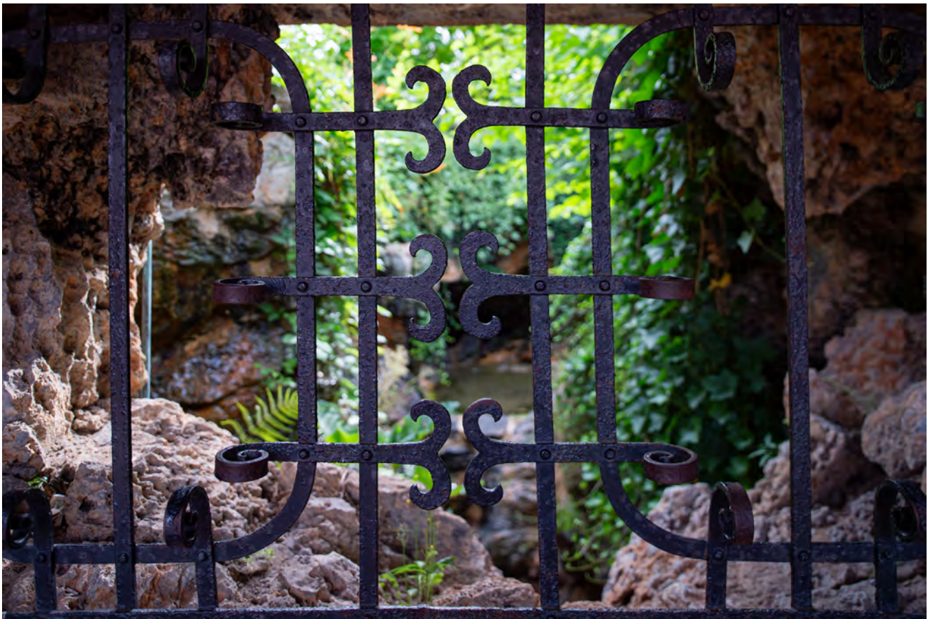
The view through the wrought-iron window grate into the lush overgrown grotto of the Summerhouse. Photo provided by AOC Photo Branch
