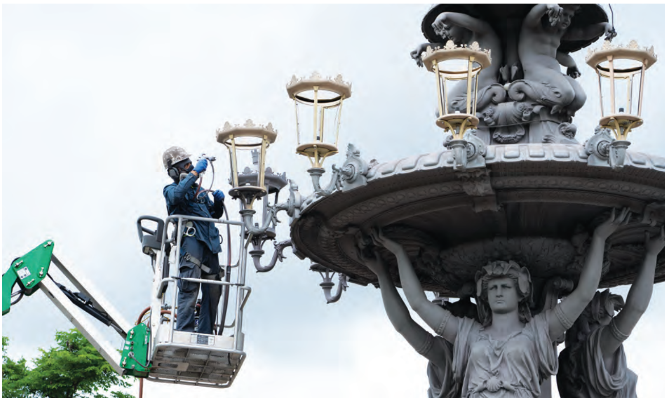
Above The AOC recoated the Bartholdi Fountain, removing deteriorated paint down to the cast iron and applying three ultra-high-performance coatings, including a Teflon-like finishing coat. The project also included a cleaning of the perimeter lampposts and the sculpture's glass lanterns.
