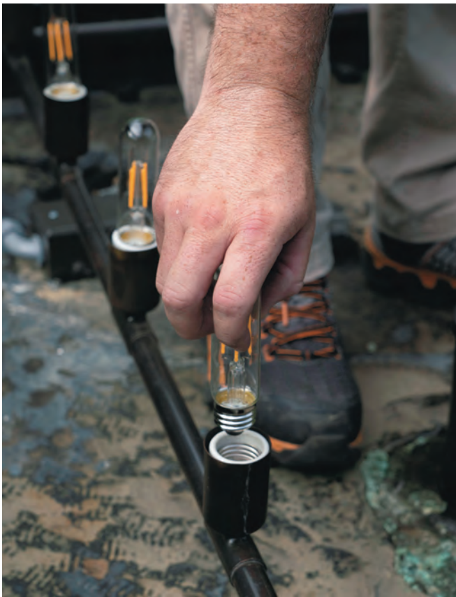
Screwing in new LED lightbulbs styled to resemble the flames of the lanterns' original gas jets.
