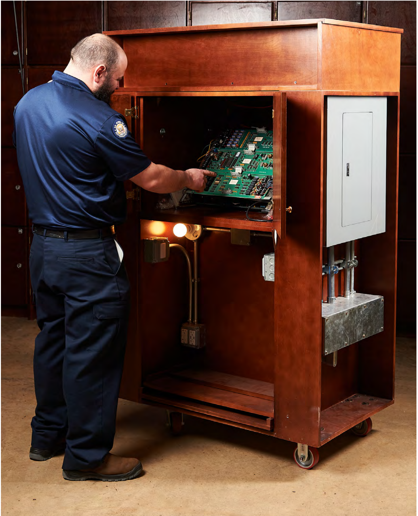
Greenwell points out the fire alarm control boards; underneath are the light bulbs and electrical switches that children played with during Take Your Child to Work Day.
