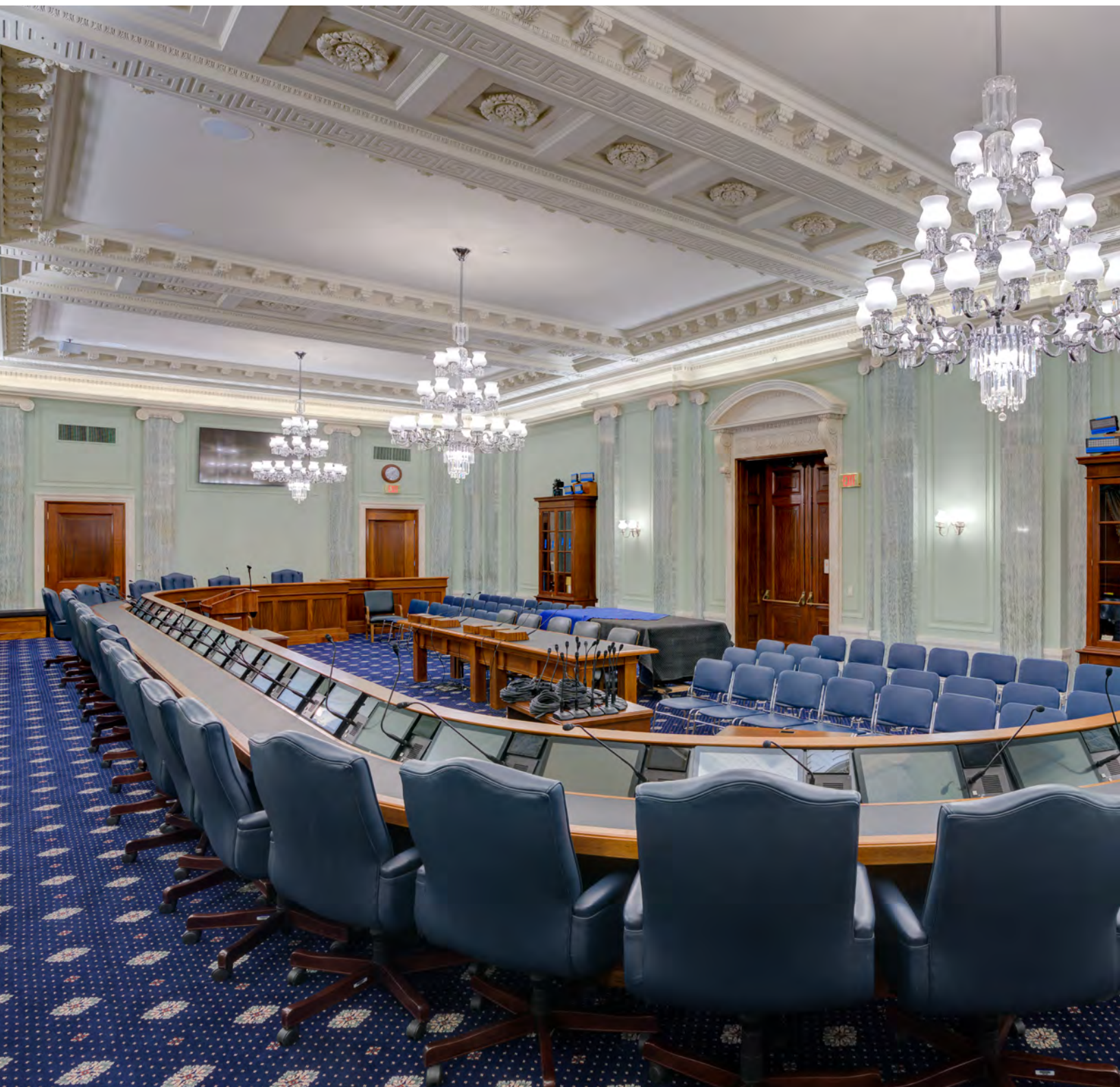
The finished SR-253 hearing room, with the ceiling and plaster reliefs repainted to appear like carved stone, which is truer to the architects' original intention.
