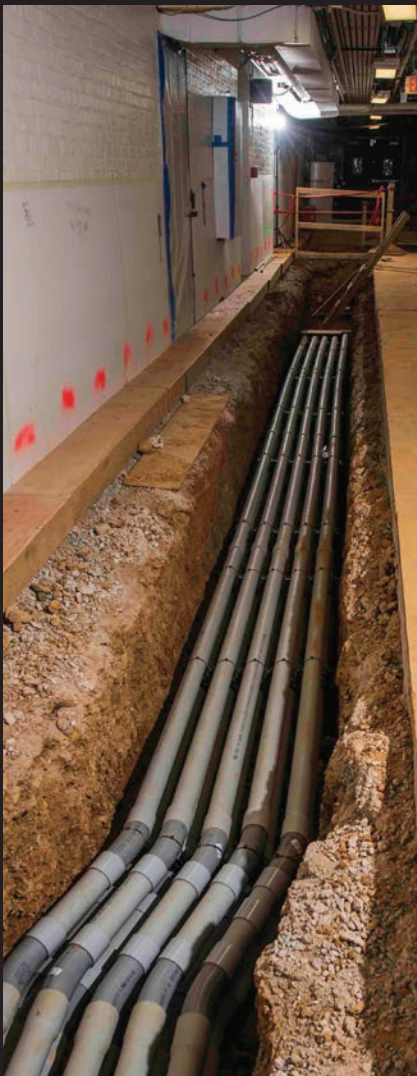
While the west basement corridor was closed, workers excavated portions of the corridor, seen here in September, to install new conduit.
