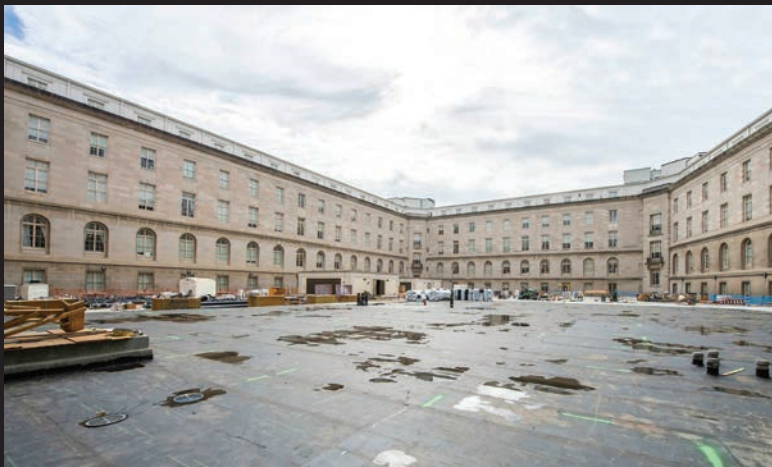
Construction crews installed concrete and waterproofing on the west side of the Cannon courtyard, seen here in October, to accommodate an eventual green roof that will be installed during the final phase of the project. The east side of the courtyard will undergo the same process starting in the spring.
