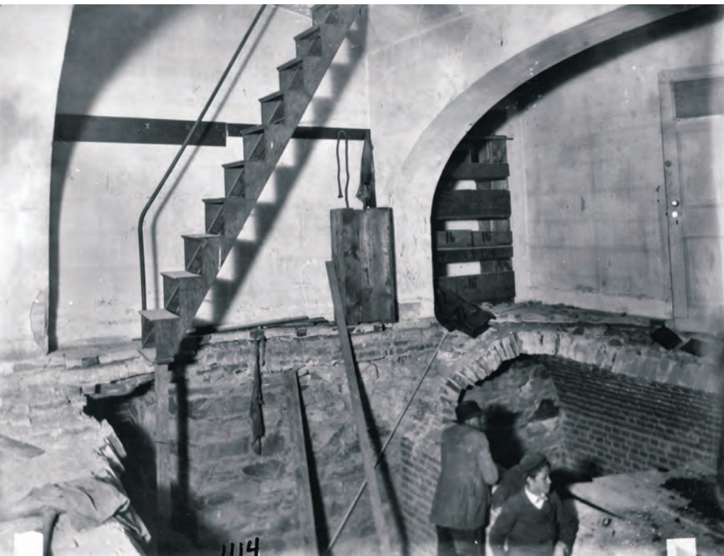
LEFT: The 1898 gas explosion blew away the stone floor in the small Senate rotunda, exposing the cellar where a fire raged until the AOC’s chief electrician crawled through the debris to turn off the gas. RIGHT: Members of the press work below a chandelier with both gas and electric lamps. Photos courtesy of AOC Photo Branch Archives
