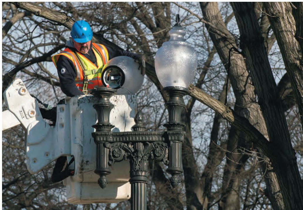
Berry Russom, High-Voltage Electrician Leader, works on a streetlight. Switching to high-efficiency lamps across the campus is one way the AOC has reduced energy consumption by 30 percent within 10 years. Photo by Susanne Bledsoe
