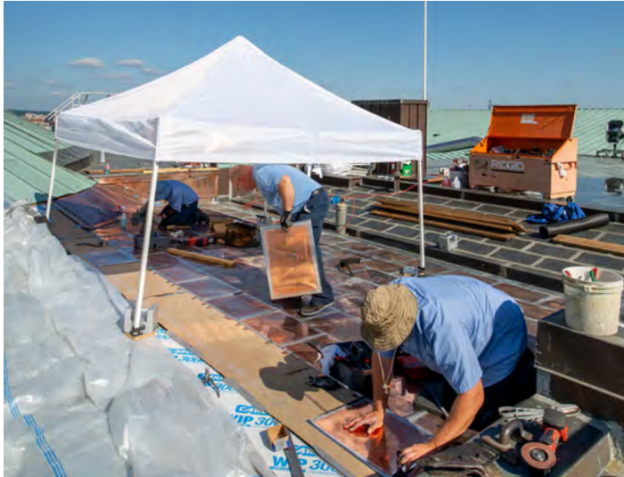
Image: Jason Stone, Brian Jerdon and Kevin Golden install flat seam copper roof panels
