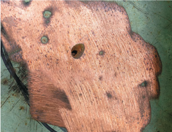
Image: Copper roofing thins over time, and when holes are found, they are patched until the section is replaced
