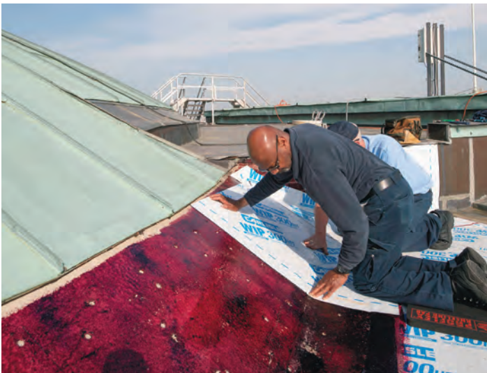
Image: Brian Jerdon installs a waterproof membrane before the copper wall flashing is placed at the base of the Senate cupola
