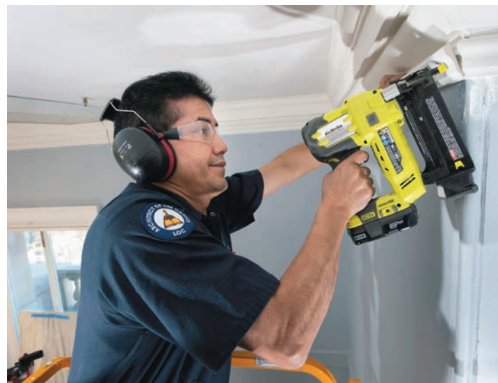
Will Guzman installs cornice trim in the Jefferson Building's attic.
