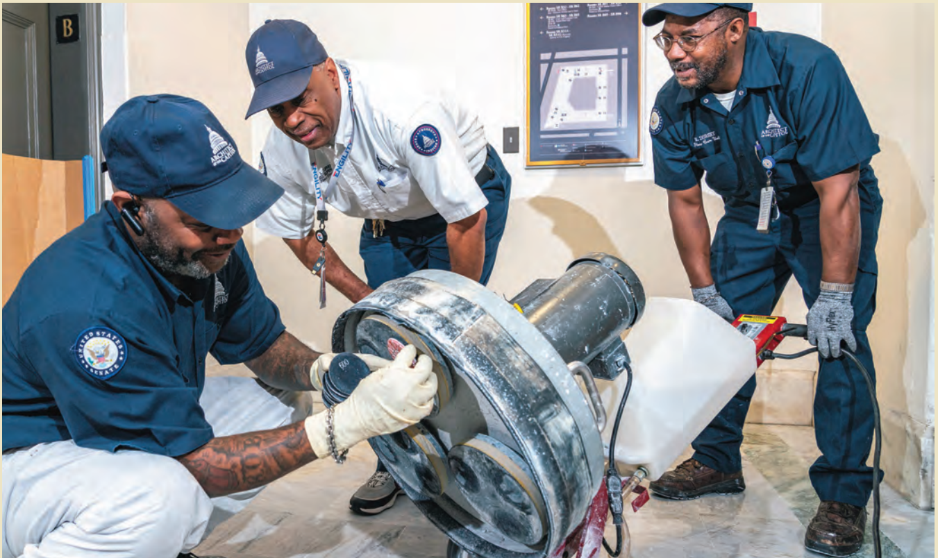
(left to right) Robert Brown, floor maintenance leader, changes the honing disks to a finer grit which contains a higher percentage of diamond particles to further smooth the stone and bring out its natural shine. Lionel Turner, floor maintenance technician assistant supervisor, and Wayne Dorsey assist with the process.
