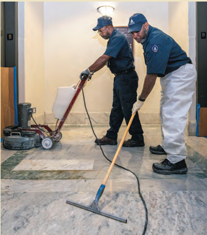
(left to right) Wayne Dorsey continues to hone the floor, while Robert Brown uses a squeegee to keep the liquid from spreading beyond the work area.
