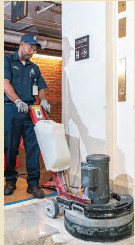
Wayne Dorsey, floor maintenance technician, hones a section of marble floor using water and a series of disks of increasingly smaller grit sizes. While the interaction between the water and the stone initially results in a white liquid known as slurry (as seen in the photo), as the natural oils from the stone start to surface, the water becomes clearer.
