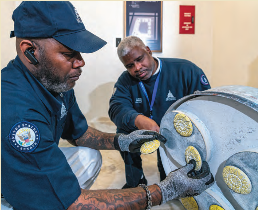
(left to right) Robert Brown, floor maintenance leader, installs resin honing disks onto the planetary head to begin restoration of a section of historic marble floor in the Russell Senate Office Building. Looking on is Dennis Anthony, floor maintenance technician supervisor.
