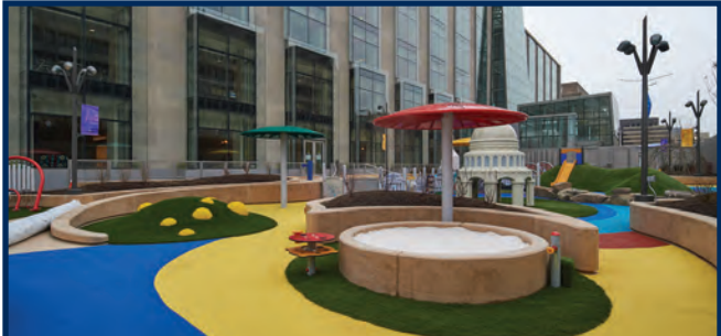
The AOC completed the first phase of the House of Representatives Child Care Center project.
