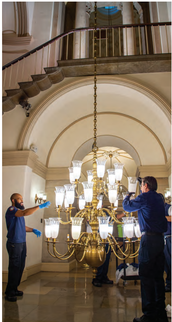
The AOC is responsible for facilities maintenance tasks — including preventive and recurring maintenance activities. One such task, shown here, is the periodic lowering of a chandelier in the U.S. Capitol Building's House of Representatives wing for routine cleaning and relamping.
