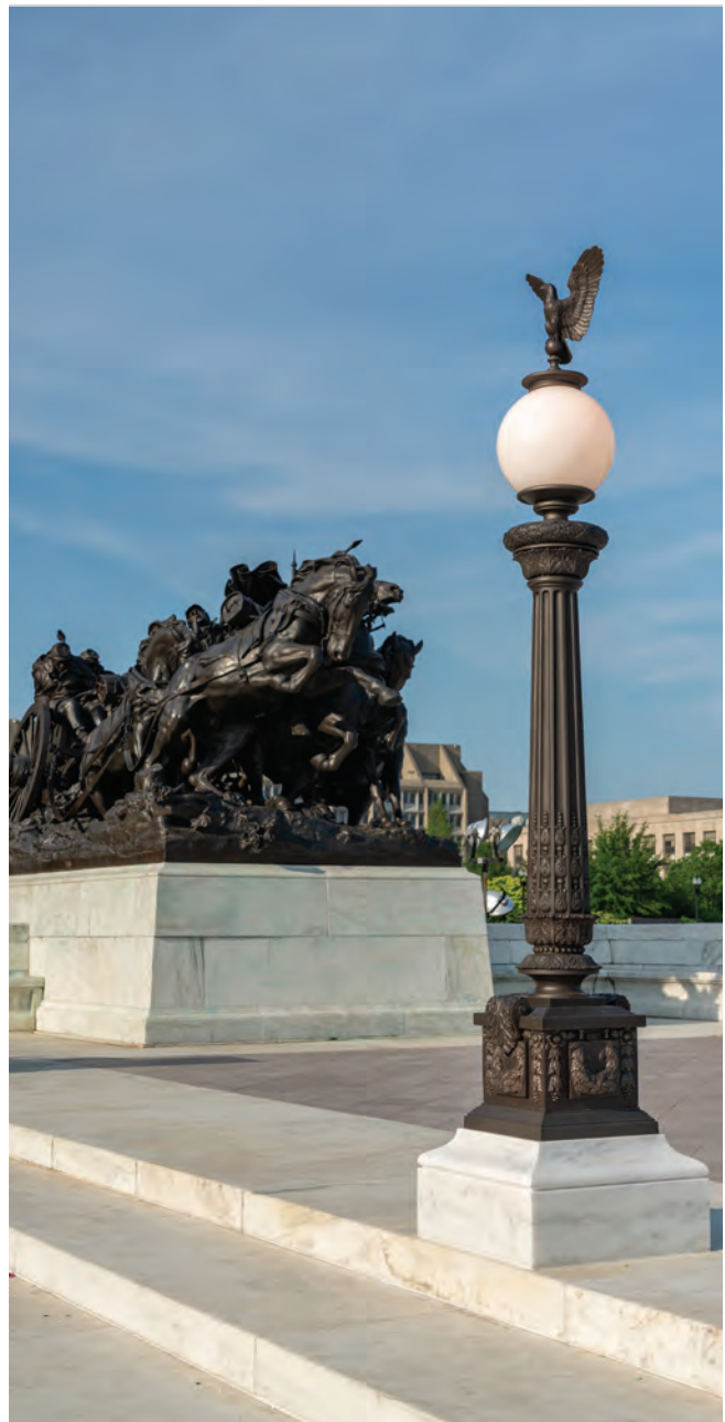
In FY 2019, the AOC conducted stone repair work on the Ulysses S. Grant Memorial and installed replica lamps.
